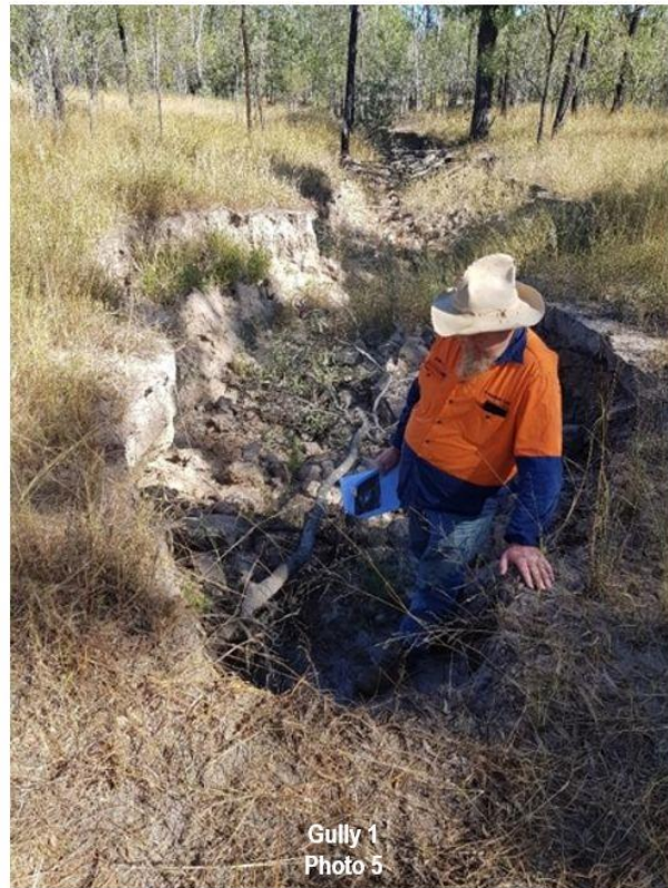
Figure 39. Gully 1 ground photographs.
